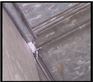
Aeroseal duct sealing technology is delivered as an aerosol mist that is blown into the interior of the ductwork. The microscopic particles of sealant remain suspended in air until they reach a leak. Here, they cling to the edge of the hole and then to other sealant particles, until the leak is completely sealed. Note that the aeroseal sealant does not coat the duct interior but accumulates solely at the leak sites.
